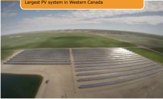
2 MW Solar Farm – Bassano, Alberta Largest PV system in Western Canada
