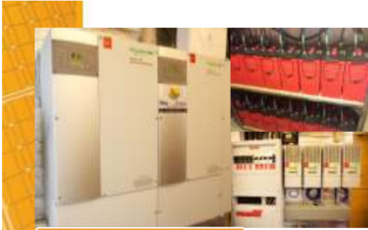
Grid tied with battery backup
